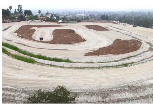
**September 2013.** The deck of the Lower Sediment Placement Site (SPS)(oak mitigation site) during mitigation site preparation. Partially distributed, salvaged native mulch is visible in the background. A large volume of mulch was incorporated into the soil via heavy equipment to a minimum depth of two feet.
