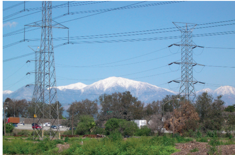
Figure 3-5. Utility easements, such as this one at the Woodland Duck Farm, offer open space area enhancement opportunities.
